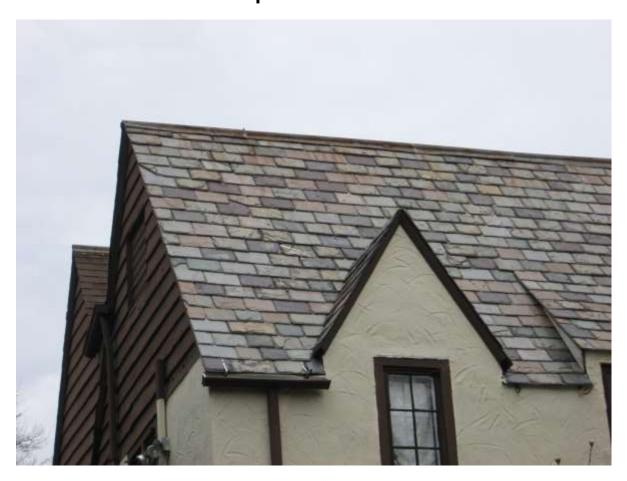
The roof system is also comprised of vents, masts, chimneys as well as the shingles. These all require a weather seal that can be copper, metal or rubber material. Over time these will all require attention. The metal flashings that keep the roof sealed to the chimney were not visible for evaluation. These areas need to be corrected as necessary to keep moisture out.
