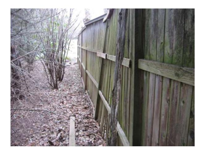
The fence sits on an interlocking wall that in places shows signs of movement over the years. It is recommended to consult a fencing company for repair and replacement recommendations.
